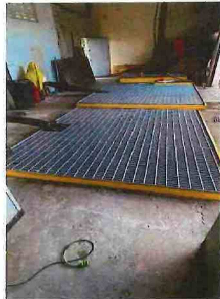
Sump safety grating was installed to improve operational safety
