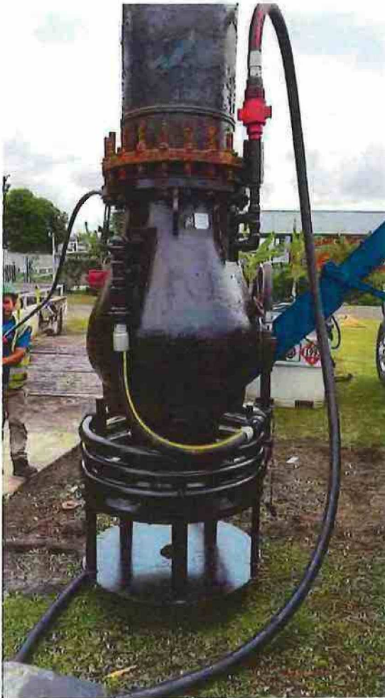
An overhauled pump unit was installed at the San Fernando Pump Station as part of the site's rehabilitation and performance recovery plan.
