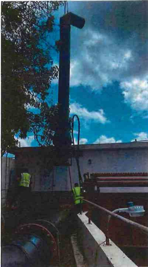
Pump Removal at San Fernando Pump Station
