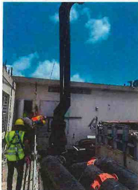
Pump Being Visually Inspected at Sabana Pump Station
