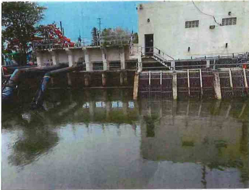
La Malaria After Pump Station After removing all debris
